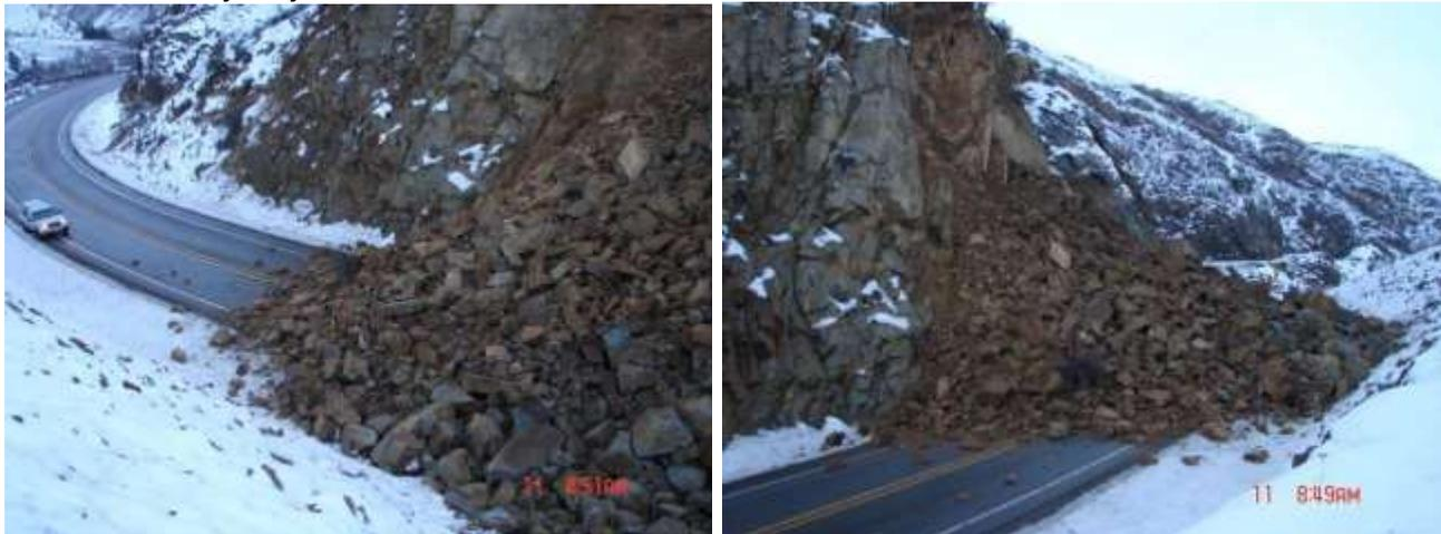
Looking at the third image, this is a complex wedge type failure on existing joints. There appears to be weathering on the newly exposed surfaces. Looking at the rest of the rock mass, the joint pattern is very complex, so this is a difficult slope to manage and mitigate.
